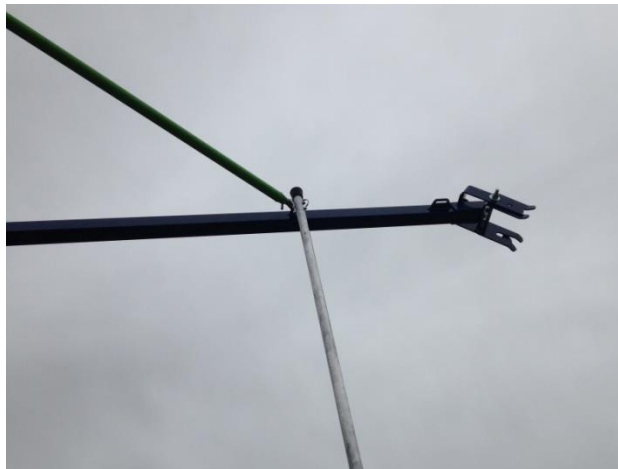
Figure 29. Removing the Brace Rod U-Clip
