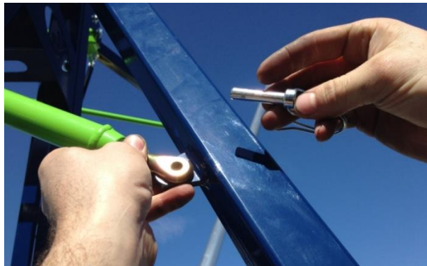
Figure 5. Lining up the Brace Rod
