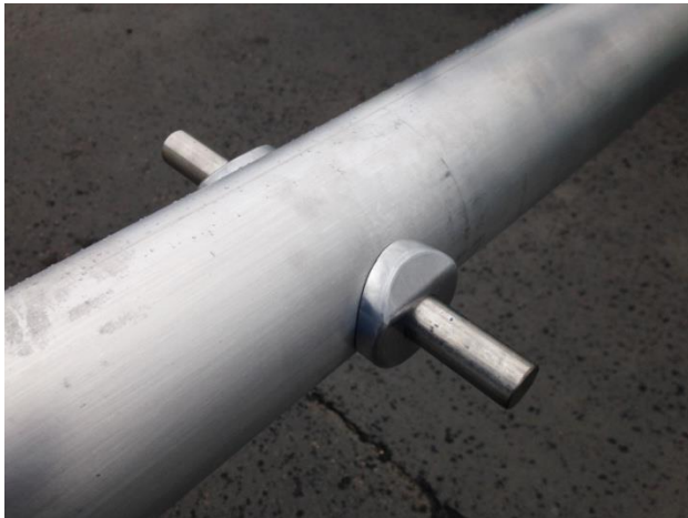
Figure 9. Beveled Edge of the Aluminum Pole
