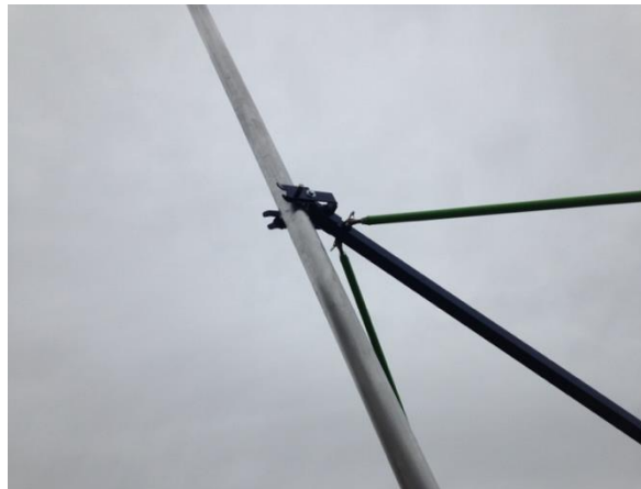
Figure 14. Locking the Poles into the Support Arms
