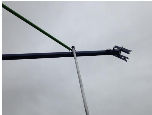
Figure 29. Removing the Brace Rod U-Clip
