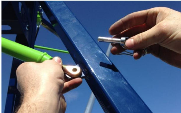
Figure 5. Lining up the Brace Rod
