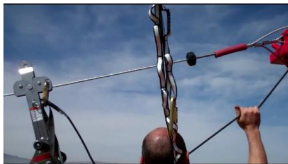
Figure 36. Tower Employee – Auto-Retract Priming
