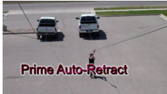
Figure 37. Ground Employee – Auto-Retract Priming
